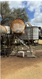
Gravity Overhead Diesel Tank 1
